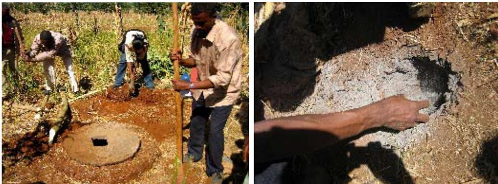
*The corner posts being dug. Ash being added to the holes before poles inserted. Soil is rammed in the holes around posts to secure.*
