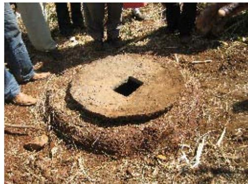
*The slab is then moved on to the ring beam so it is supported equally all round. It is bedded in so the slab is well supported all round.*
