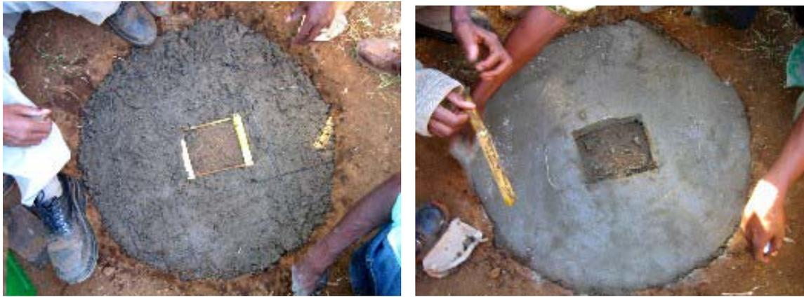
*The wooden squat hole frame is removed and the edges of the hole are made neat with a trowel. Wire handles can be added, but with small slabs they are unnecessary. The slab is made neat and smooth using the steel trowel.*
