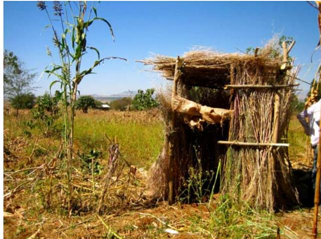
*The fifth post is added in between the two front posts and half of this is also filled with walling material. The opening is for the door which can be covered with a cloth hanging down from the upper beam. A simple door on rubber hinges (car tyre etc) can also be added.*
